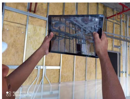
Fig. 5. Implementation of Augmented Reality Technology in Construction: Site engineer utilizing tablet-based AR interface to overlay BIM models onto the physical construction environment, enabling real-time collision detection and enhanced visualization during the installation phase.
