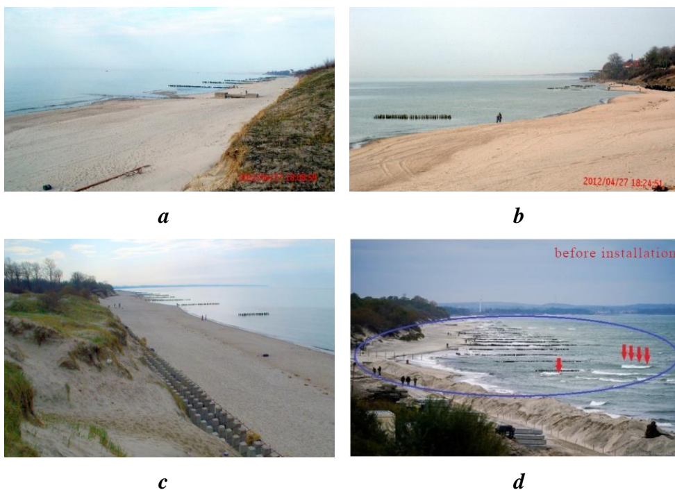
Fig. 2. State of the beach: a – stable beach at the western tip of the old groins site (the early 20 th cent.) (27.04.2012); b – lee erosion at the eastern tip of the old groins site (27.04.2012); c – seasonal beach restoration identified by a strip of washed sand, including in the shady zone of the groins (27.04.2012) (photo by A. N. Babakov); d – the state before the period of autumn-winter storms in 2020, 19.10.2020. The arrows indicate the future position of the breakwater modules
