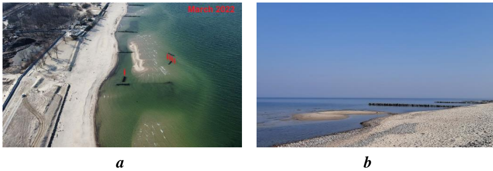
Fig. 12. Exposure of the top of the underwater alongshore bar in March 2022 shortly before its attachment to the water's edge at an extremely low sea level: a – the shore segment where the breakwater was installed (red arrows); b – the shore segment 400 m west of the breakwater installation site
