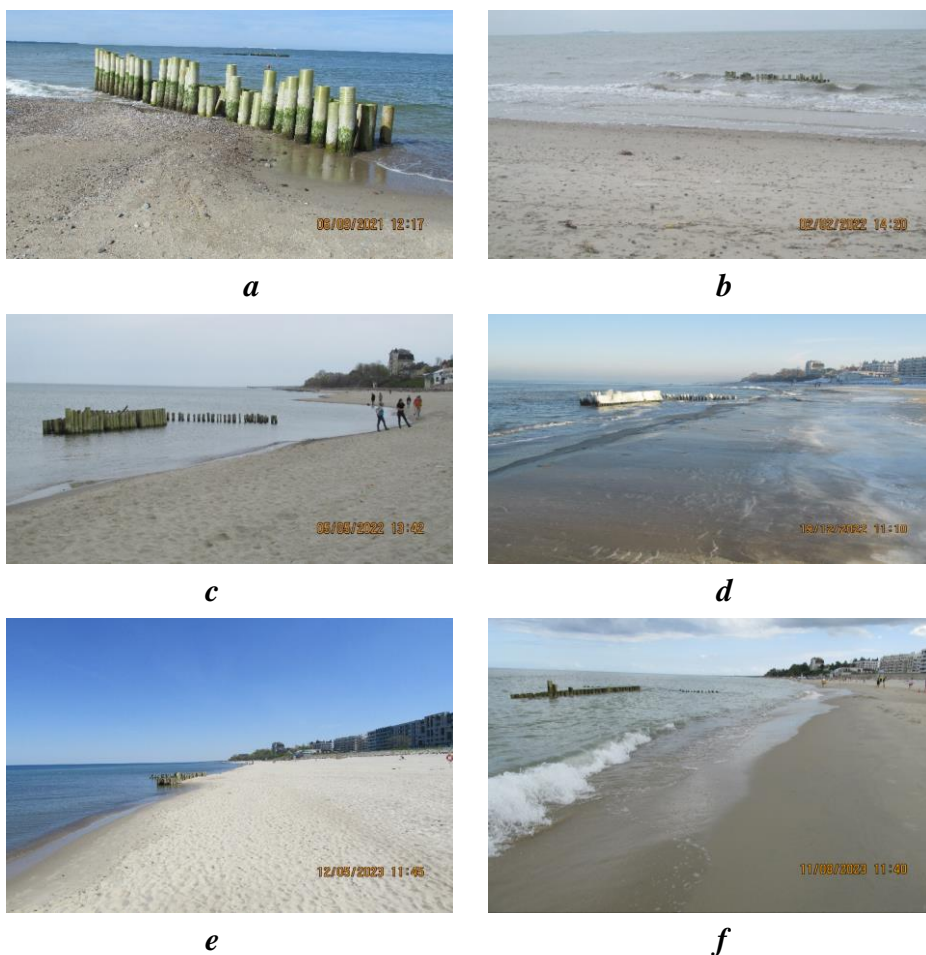
Fig. 4. The beach dynamics after the installation of the breakwaters in 2021–2023: a – summer accumulation, 06.09.2021; b – beach narrowing after extreme storms, 02.02.2022; c – the state of the beach after the storm period, 05.05.2022; d – beach nourishment in the finishing phase of the winter storm, 19.12.2022; e – the beach restored by moderate spring waves, 12.05.2023; f – beach narrowing due to a noticeable increase in the sea level, 11.08.2023. Photo by A.N. Babakov
