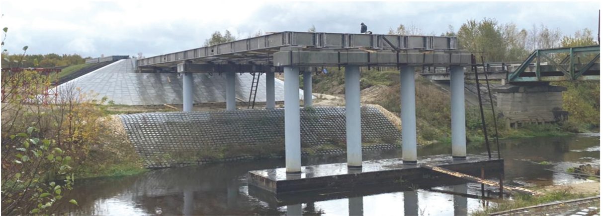
Fig. 17. Installation of the span on reinforced concrete supports
