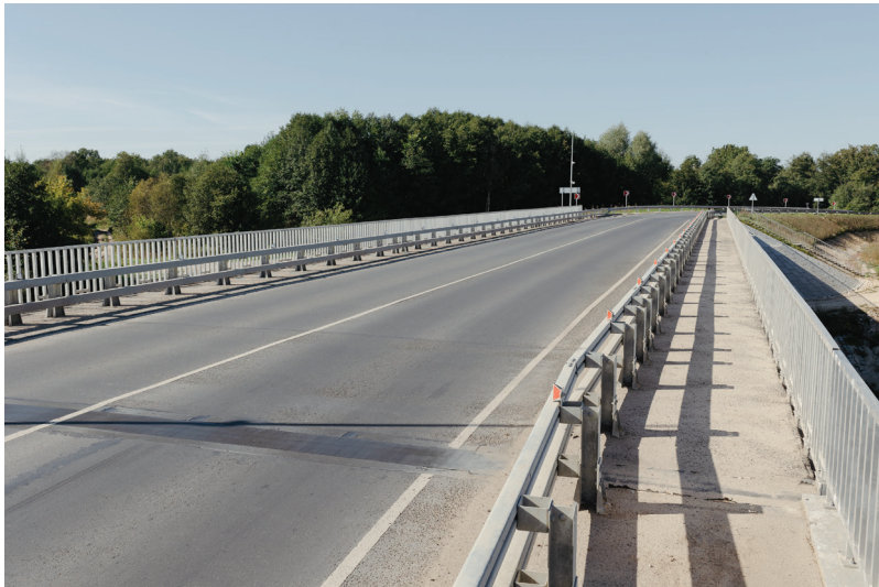
Fig. 3. View of the bridge from the side of the shoulder of the two lane highway
