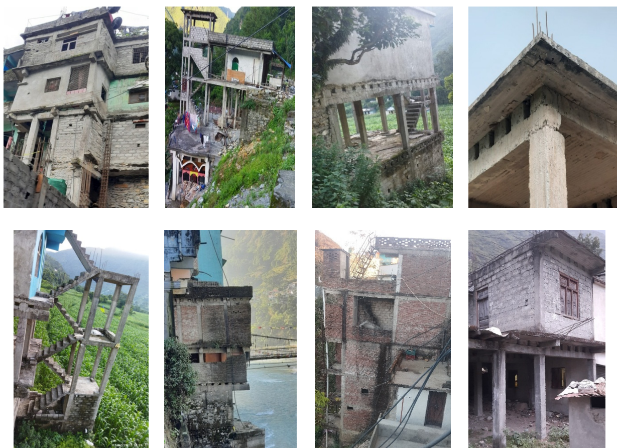
Figure 1. Non-code-compliant RC buildings observed in Darchula and Hillside
