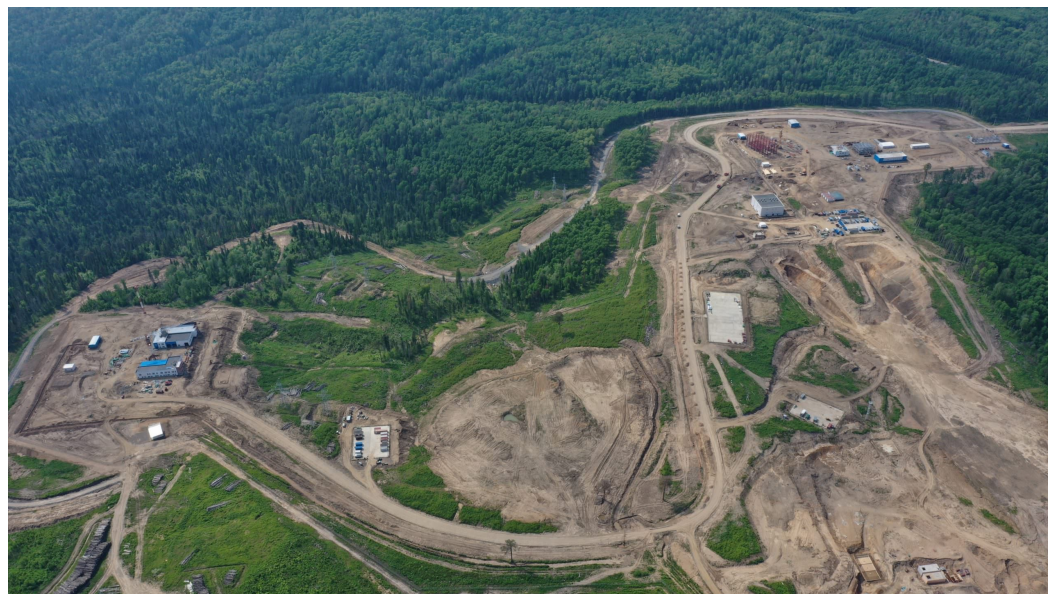
Figure 5. Construction of the underground research lab in the Nizhnekansky massif for monitoring the disposal of highly radioactive waste ( https://strana-rosatom.ru/ ).
